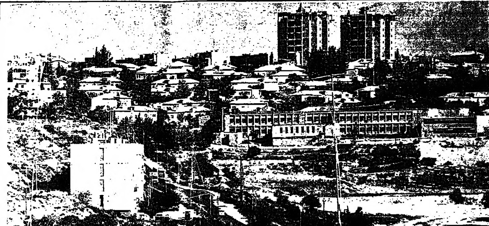
The view of Shikun Ovdim's nearly completed towers in Jerusalem's Kiryat Hayovel, as seen from the nearby area of Manahat (Malcha). The zoning of the plot, in the midst of one-storey villas, was changed from "public" (for schools or parks) to "residential" to accommodate the project. The City Engineer's Office now reports that Shikun Ovdim has asked permission to build two more towers across the street from these, but was turned down on aesthetic considerations. Jerusalemites are asking where the aesthetic considerations were when the first two buildings were permitted. And where are the parks? (Rubinger)
